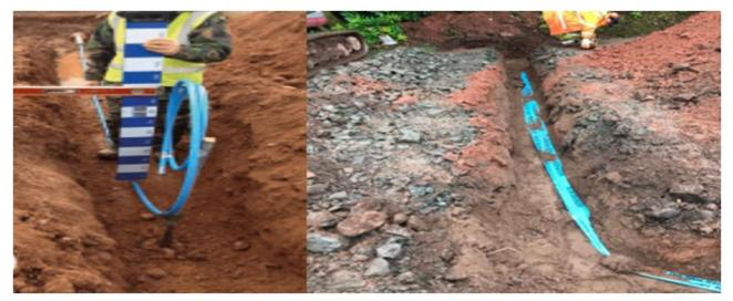
Track with sand, pipe and marking tape laid above. This should be a minimum depth of 750mm, and Marker tape should be laid at a 100mm-300mm above the supply pipe for the whole length of the track.
