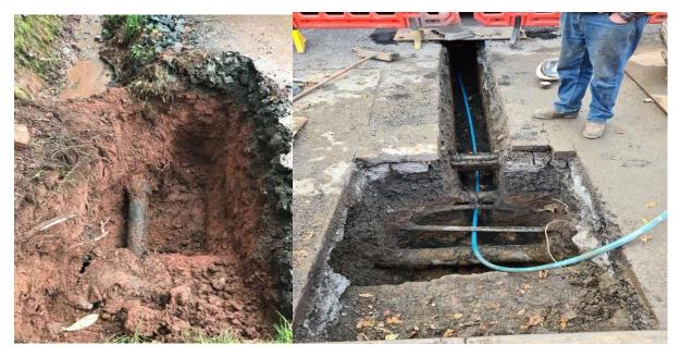
Exposed water main for connection – excavation should be approx. 1m x 1m and 150mm clearance below the main to allow for the connection. A measuring stick /tape should be used to show the depth of the main to the finished ground level to allow for safe access/egress from the excavation.
