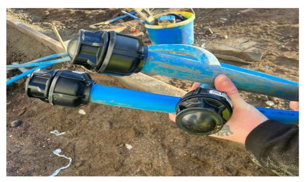
The supply must be capped off with either a plastic cap or a Philmac fitting and must be shown in the photo above.
