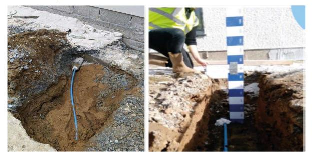
Point of entry – showing insulated supply pipe going through 100mm blue duct at minimum depth of 750mm. Duct should also be sealed with expanding foam.
