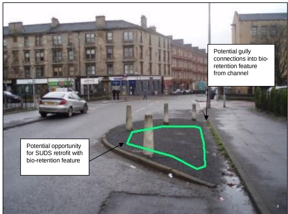
Figure 5.2 SUDS Retrofit in Road Build-out, Glasgow
