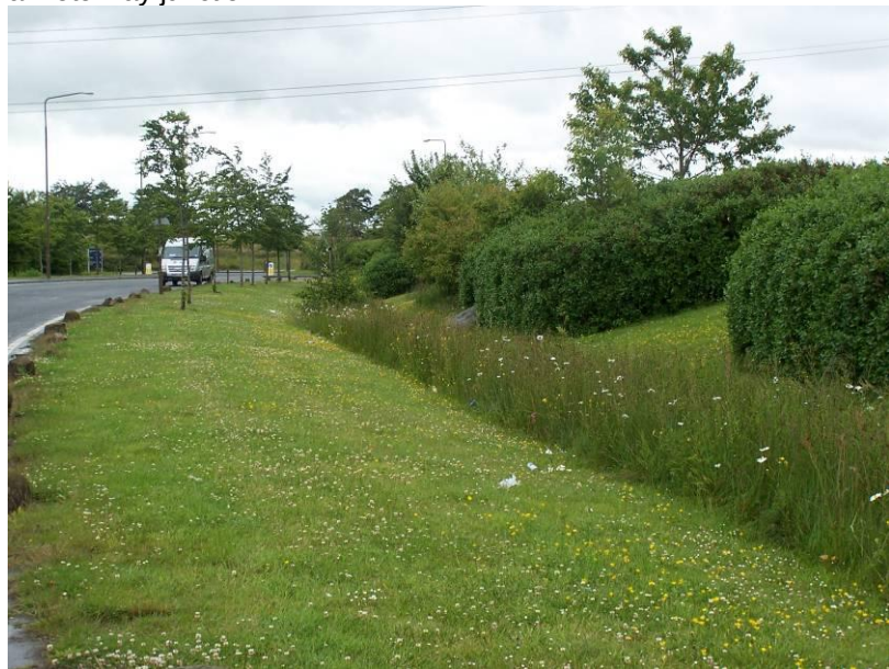
Photo 9. Filter Strip and Swale
