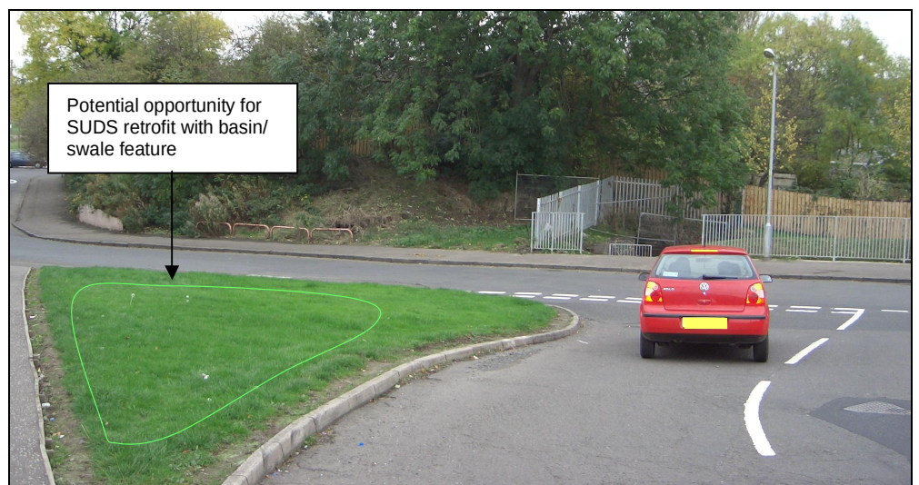
Figure 5.5 SUDS Retrofit at Junction, South Lanarkshire
