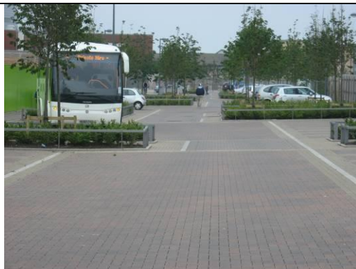
Photo 2. Permeable block paving on the site
