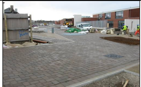
Photo 5. Road Construction Type M2 Completed
