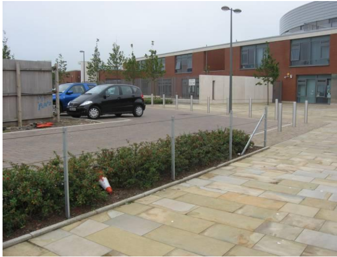
Photo 6. . Different Types of Paving Used on Site.
