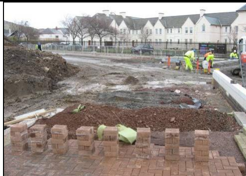
Photo 4. Road Construction Type M1 in Progress
