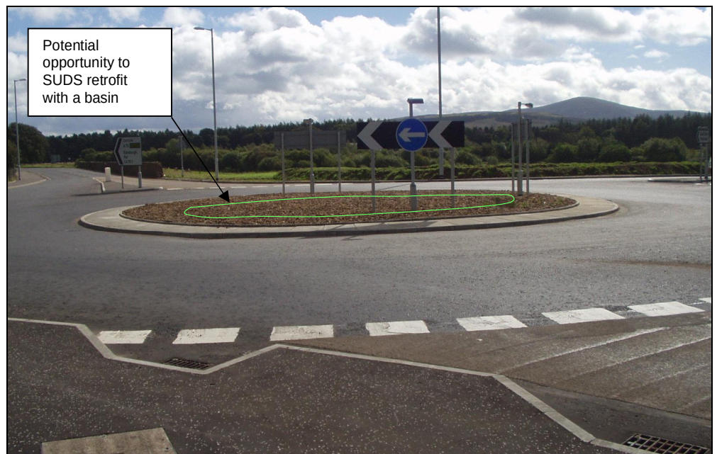
Figure 5.4 SUDS Retrofit in Roundabout Island, Lanark
