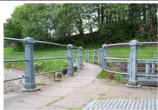
Iron rails & posts around basins and causeways
