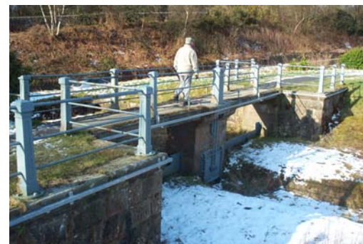
Mugdock Weir & bridge
