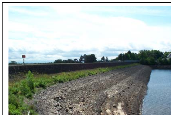
Main Causeway Revetment
