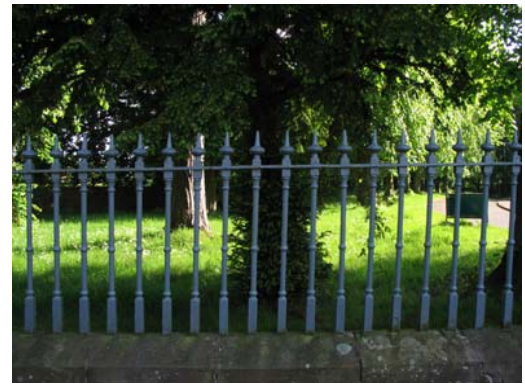
Railings at Water Works
