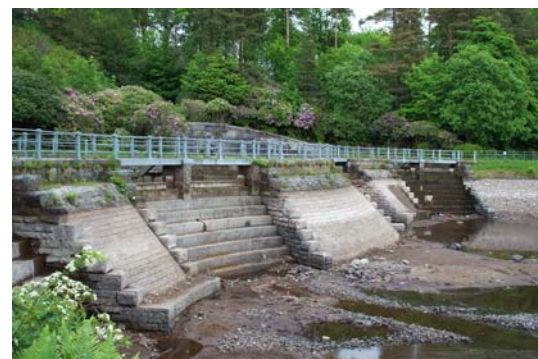
Mugdock Reservoir Gauge Basin weirs
