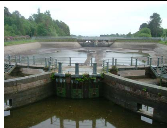
Mugdock Gauge Basin walls
