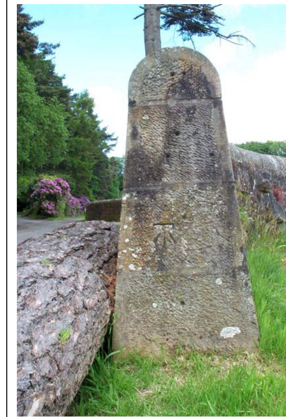
Masonry Walls – Craigmaddie Measuring Pond Causeway
