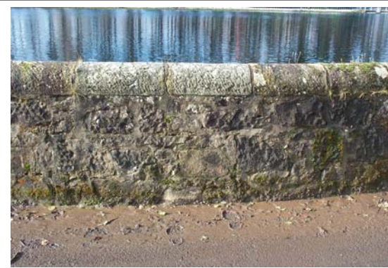
Mortared walls with half round copes
