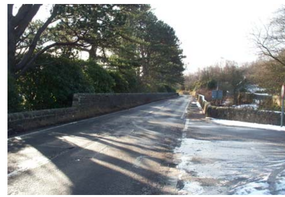
Perimeter walls (Mugdock Road)
