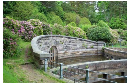
Mugdock Reservoir Gauge Basin headwalls
