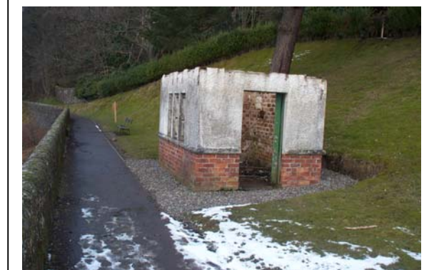
Redundant small buildings
