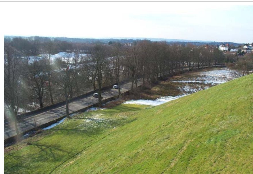
Strathblane Road Tree Avenue
