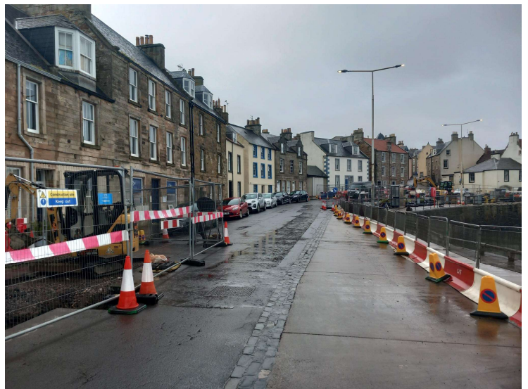
Image: Ongoing East Shore Works
