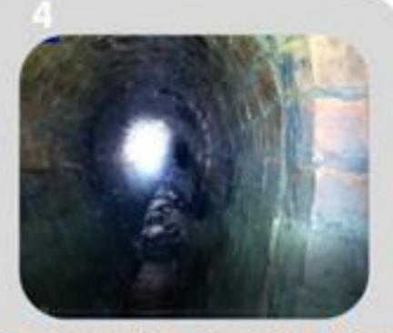
The sewer is accessed from a manhole and a camera survey is undertaken
