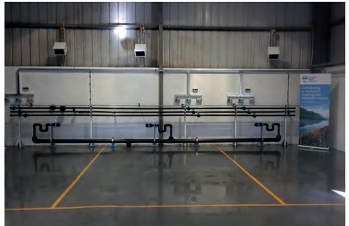
Testing bays at the Bo'ness Development Centre, showing the three different waste water feeds and the pipework to return final effluent to the adjacent treatment works inlet
